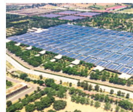
World's largest rooftop solar system at Radha Swamy Satsang Beas, Punjab
