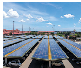
India's largest carport installation in Pune
